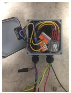
Lift the cover off the control box carefully to avoid disconnecting any wires.
